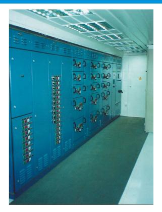
Front side view of the draw-out type panel-switchgear 400/231V for technological consumers. High wattage consumers are located in drawers (middle part of the switchgear) and low wattage consumers - on montage plates (left side of the photo)
